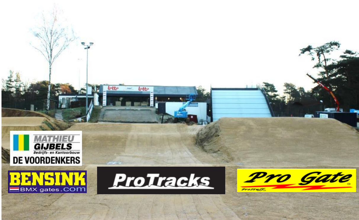
(track 5m/ 8m starting ramp Construction november 2013)
